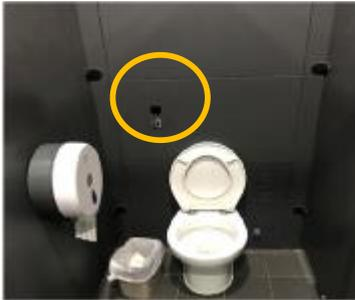
All pipelines and cables should be installed in a concealed manner. Corners with sharp angles or edges should be avoided. Opening on pipelines and access panel should be provided for maintenance purposes.
