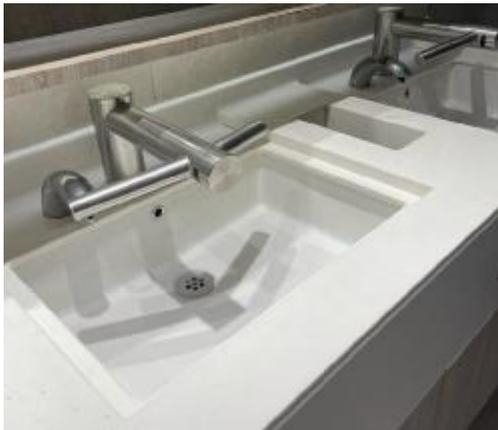
All taps for the wash hand basins should have electronic sensors. An electronic sensor soap dispenser should be fixed near the basin. A fast hand dryer is preferable instead of paper towels for drying hands after washing. An opening for a rubbish bin under the counter top is ideal for users to minimize the chances of wetting the floor while their hands are wet after washing.
